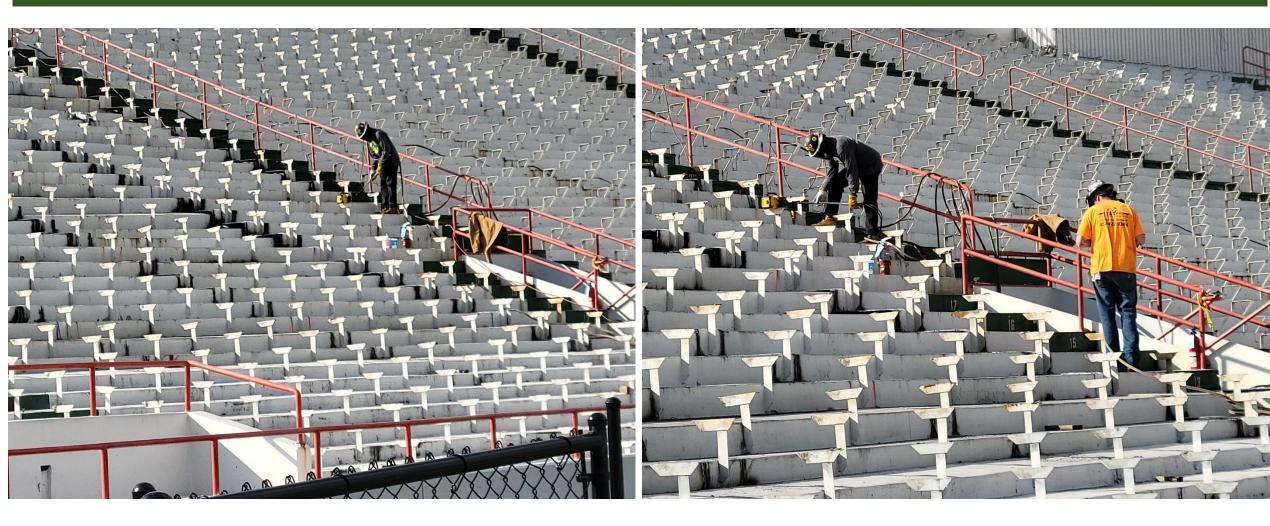
• Subcontractors cutting existing steel pans to be removed by Crane.
