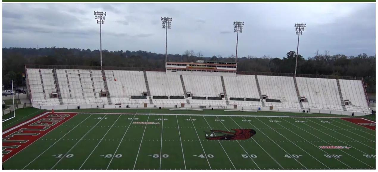
Existing westside grandstands first two sections of the stadium steel pans has be cut from structural support to be removed by Crane.
